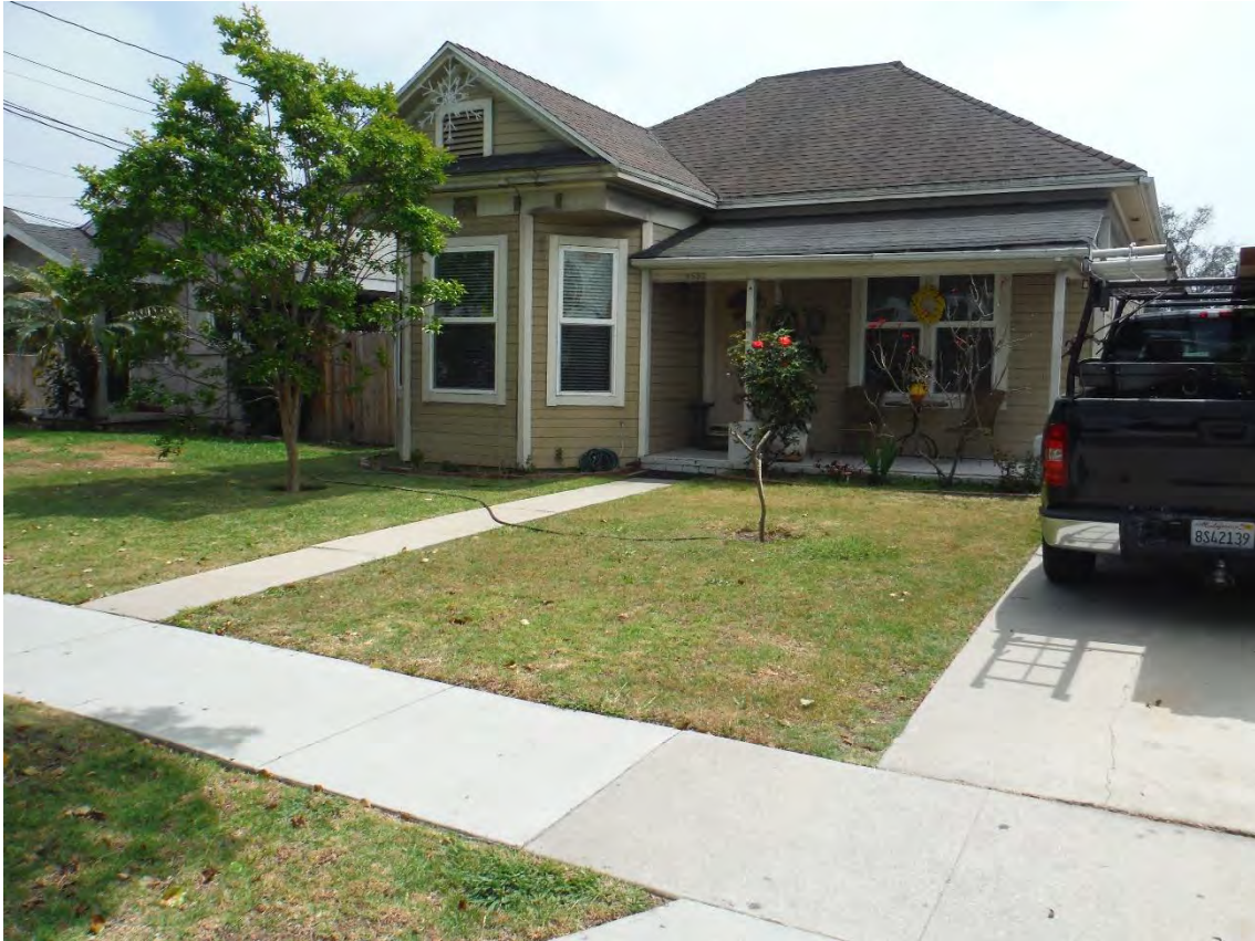
Figure 7. Single Family Residence at 4555 171 st St., view north
