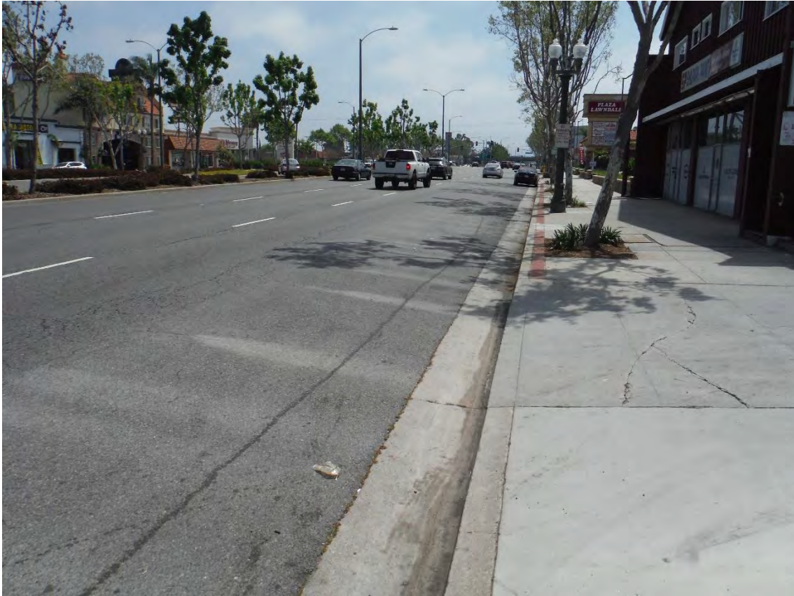
Figure 2. Project area overview along Hawthorne Boulevard, view south.
