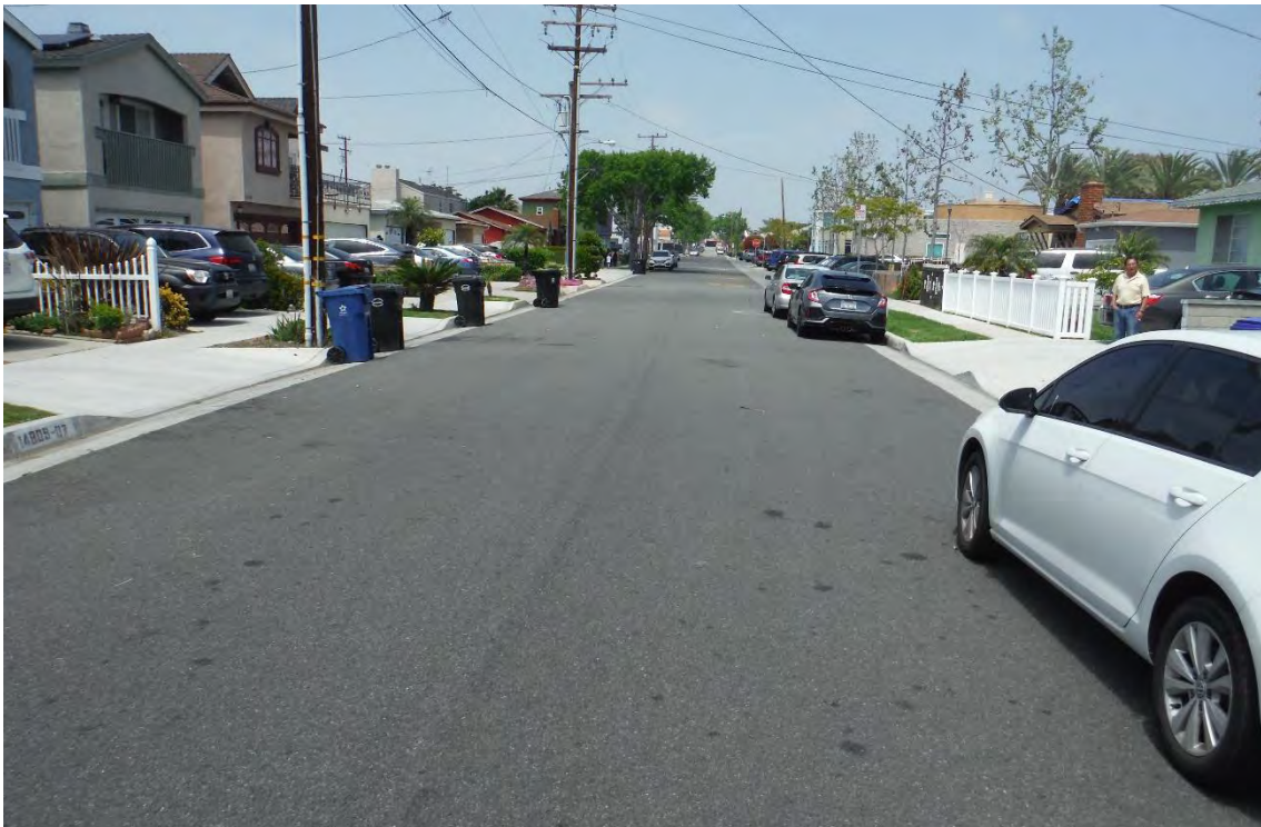
Figure 1. Project area overview along Grevellia Avenue, view north.
