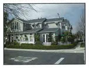
Multiple massing and second story setbacks help create varying rooflines and facades.
